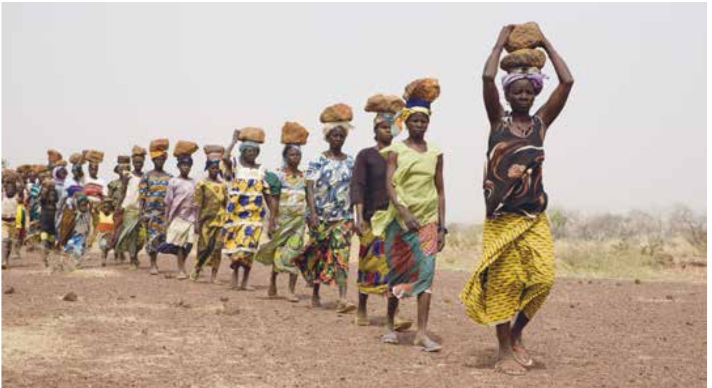
Women in Keleguem village, north-eastern Burkina Faso, carry rocks with which to build rock belts – low walls that help to protect the soil from rain and wind erosion. Built with support from Christian Aid partner Réseau MARP, the walls help crops to grow and yield more food.
