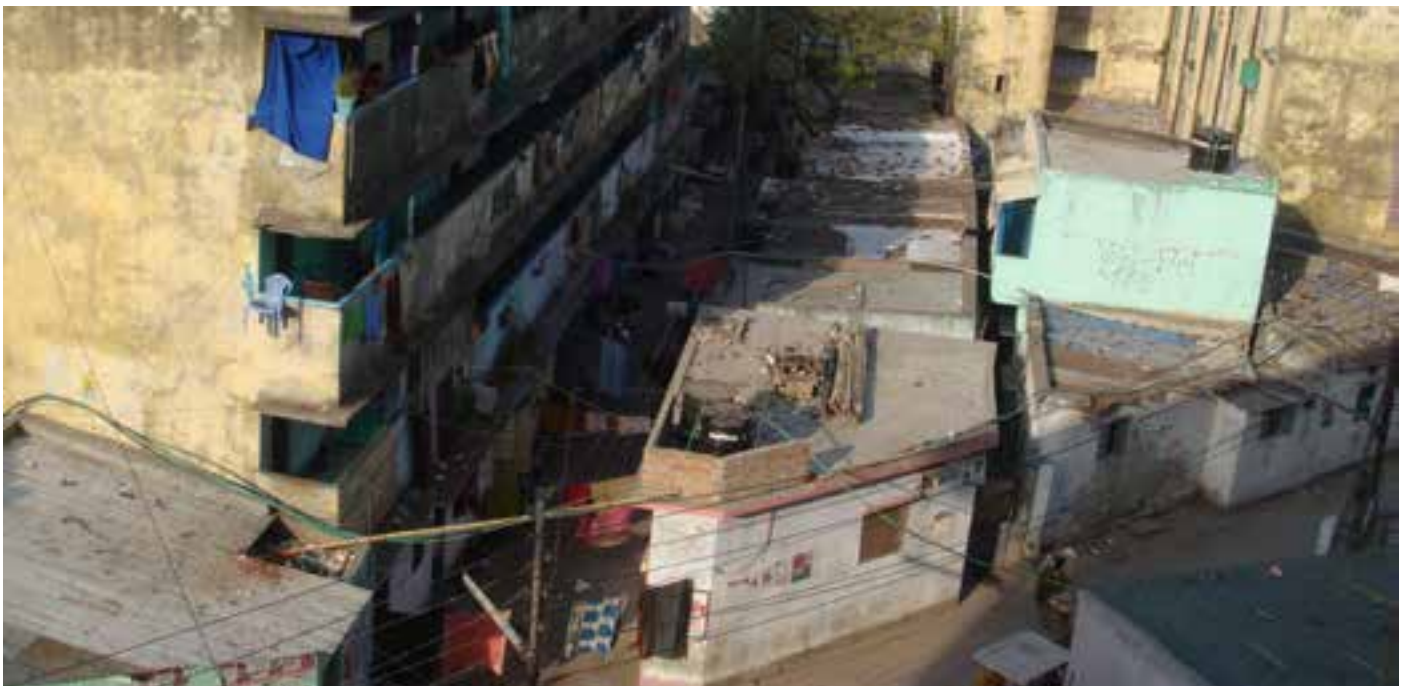
Congested living in an old multi-storey building and other types of accommodation in Dhaka City Corporation cleaners' staff residential area at Gonoktuli Lane, Azimpur, Dhaka
